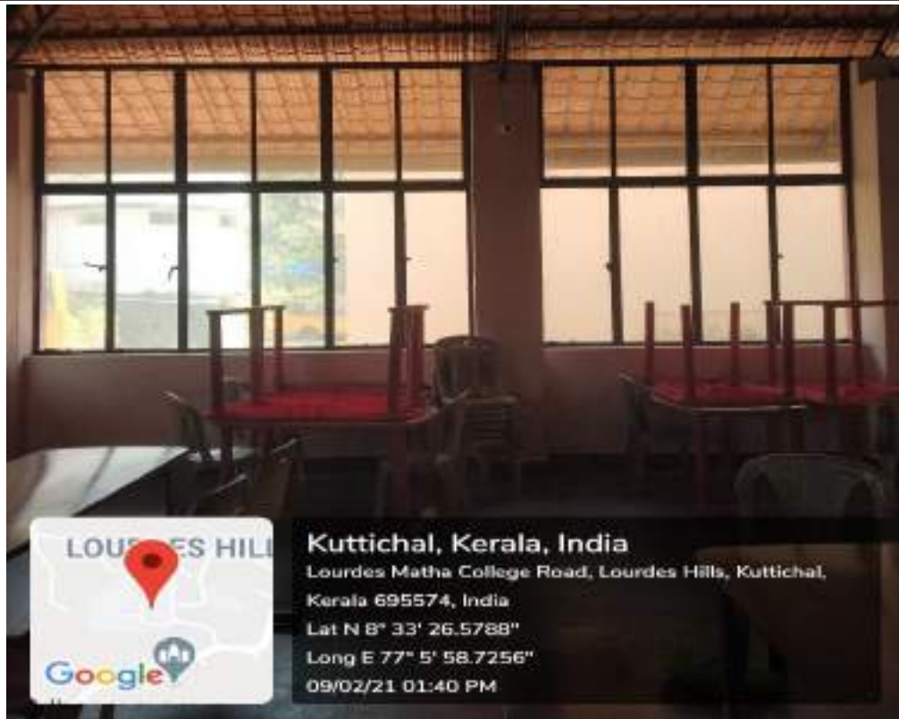
CCTV camera placed inside Boys dining hall
